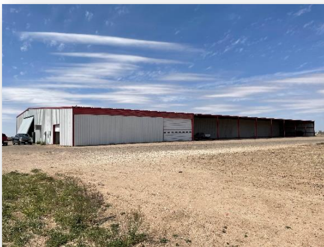
Exterior Photographs of the North Metal Building
